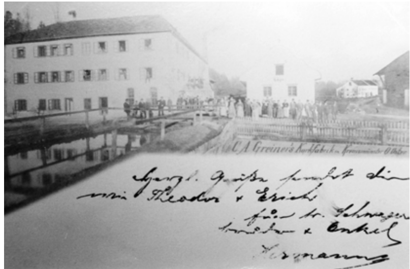
The Schaffermühle in Kremsmünster (Austria), the foundation stone of today's group headquarters.
